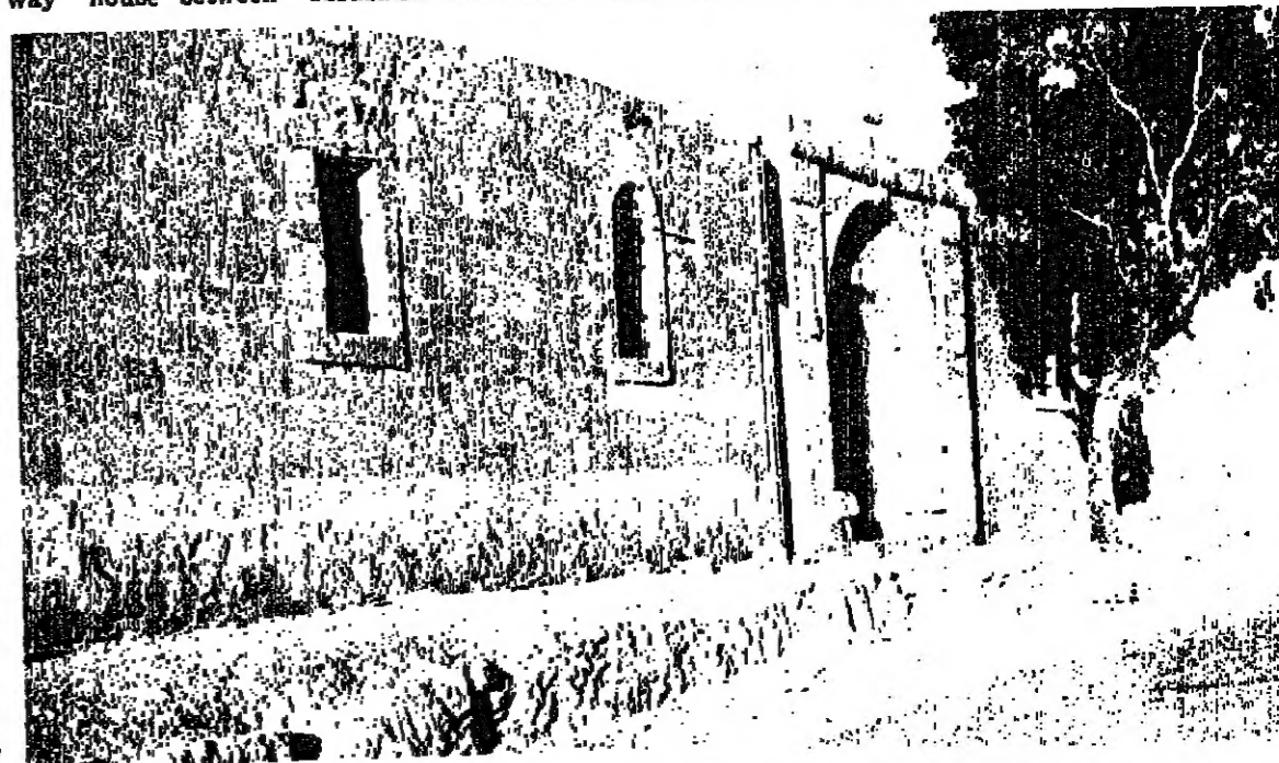
Inn building, which was used as a Turkish police post about the turn of the century.
